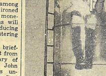
Looking like a swizzle-stick in a giant-size highball, Melvyn M. Maki is shown demonstrating the navy's new submersion suit which will enable its wearer to spend as many as three hours in freezing water.
