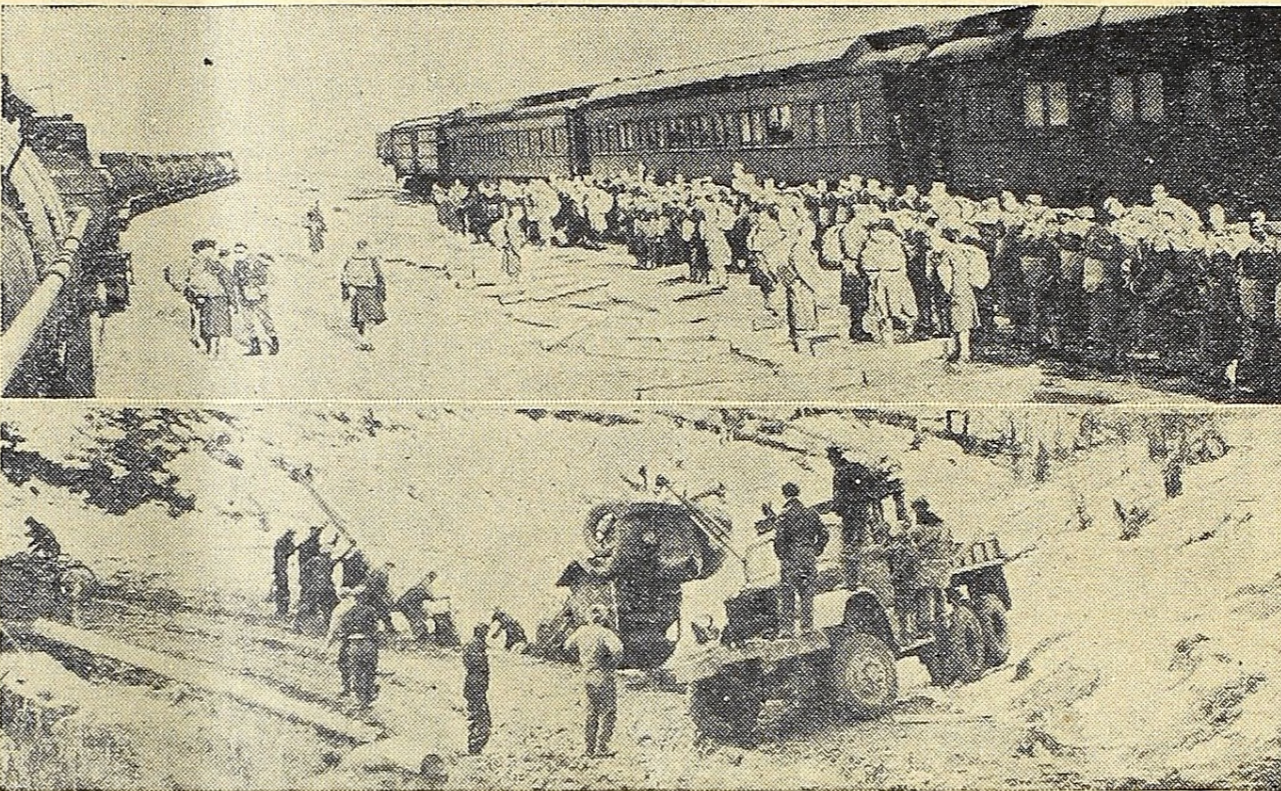
Upper picture shows journey's end, as U. S. engineer corps troops arrive at the end of the steel ribbon, at Dawson Creek, B. C., to start building a highway to Alaska from the end of the present road at Fort St. John. Below: First activity of road building at start of construction of the Alaska highway. Note men in foreground with truck pulling another road-building truck out of a ditch. All equipment for the project was shipped from the States.
