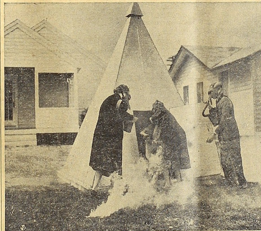
Mass production air raid shelter, shown during a tryout in Boston. It is bolted on a concrete base. Ventilation comes in at the top where the little cone crowns the steel pyramid. Yes, this shelter can accommodate 12 people. With air raid alerts on both coasts, interest in shelters is increasing. Some can be bought for as little as $200.
