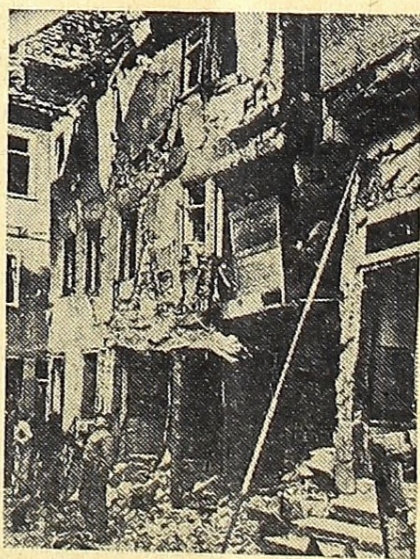
A rare picture, passed by the German censors, showing some of the extensive damage caused by raiding planes of the RAF on the residential section of Wurtemberg, Germany.
