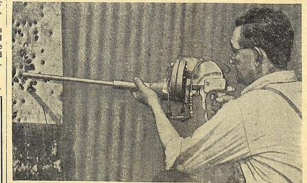
Put tarough a test by its two inventors, William Hale and Durand Beam, this rifle fired 10,000 shots per minute-with absolutely no noise. The rifle operates with compressed air. It reduced three-inch oak planks to kindling and turned airplane armor plate into steel mosquito netting. It of agriculture. A nomination by the resembles a sub-machine gun, and when it starts firing the barrel gets President is tantamount to appointcooler instead of heating up.
