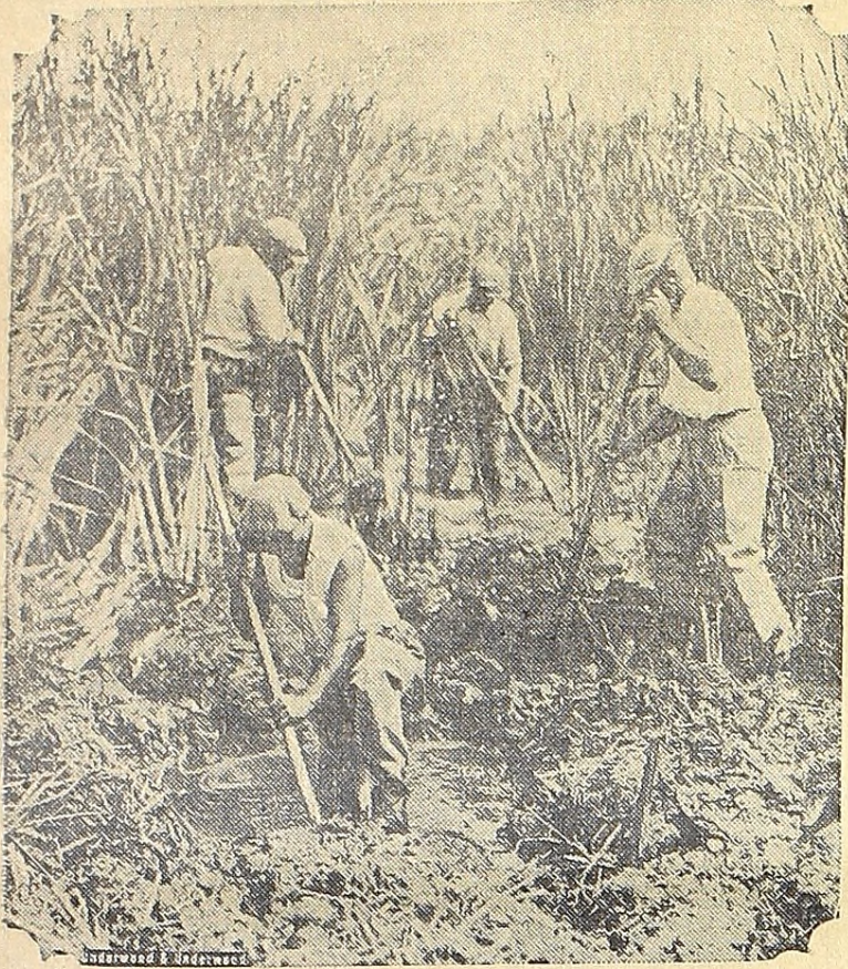
Greater New York is waging warfare on mosquitoes along a 650-mile front and has resorted to trench methods of fighting. The photograph shows workmen in the Corona marshes preparing the way for the trench diggers, who are followed by the spreaders of oil.
