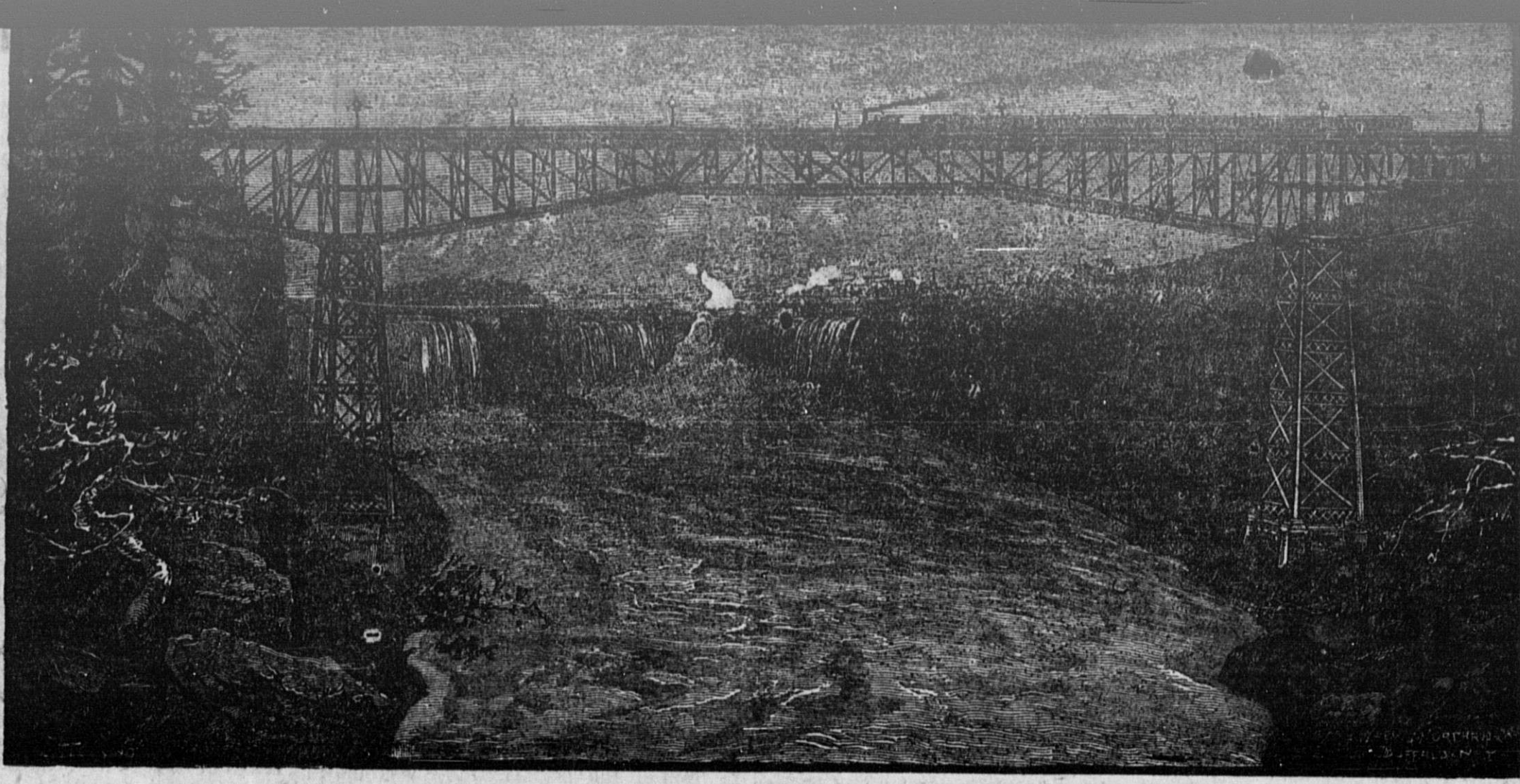
THE GREAT CANTILEVER BRIDGE.
