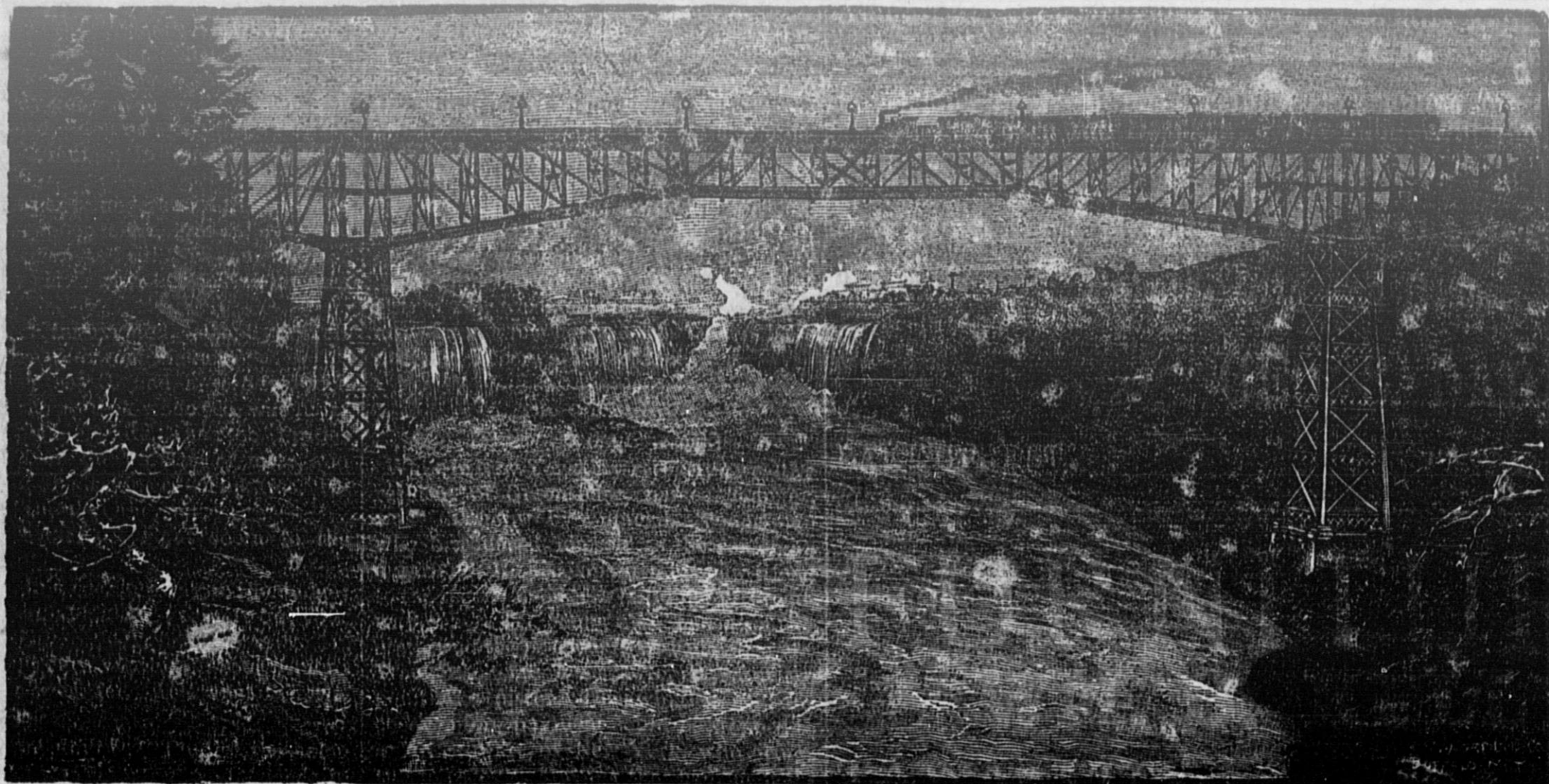
THE GREAT CANTILEVER BRIDGE.
